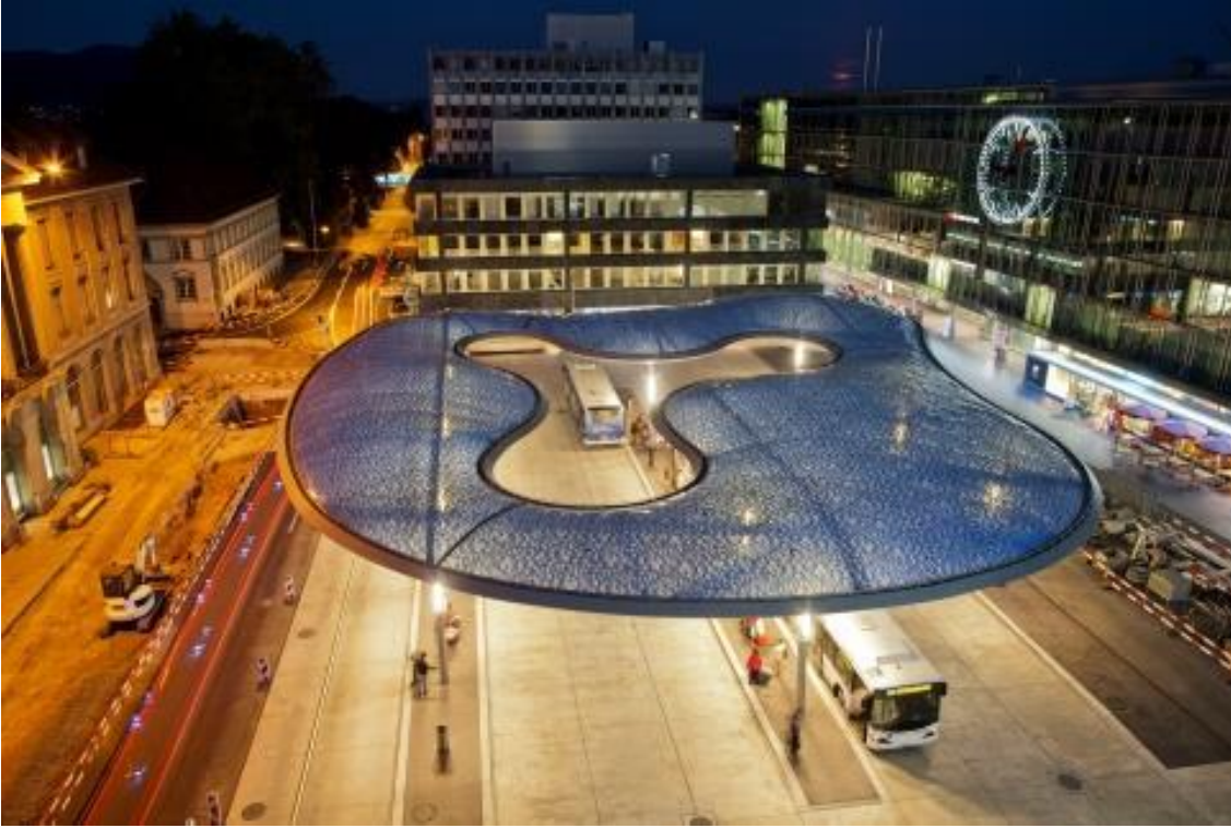
Figure 3: Bus Terminal Aarau [Niklaus Spoerri Zürich]
