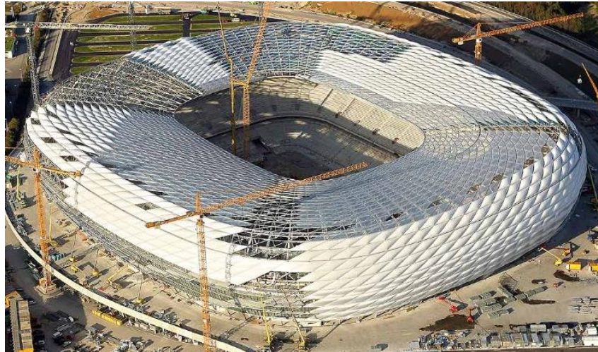
Figure 12: Allianz Arena Munich
