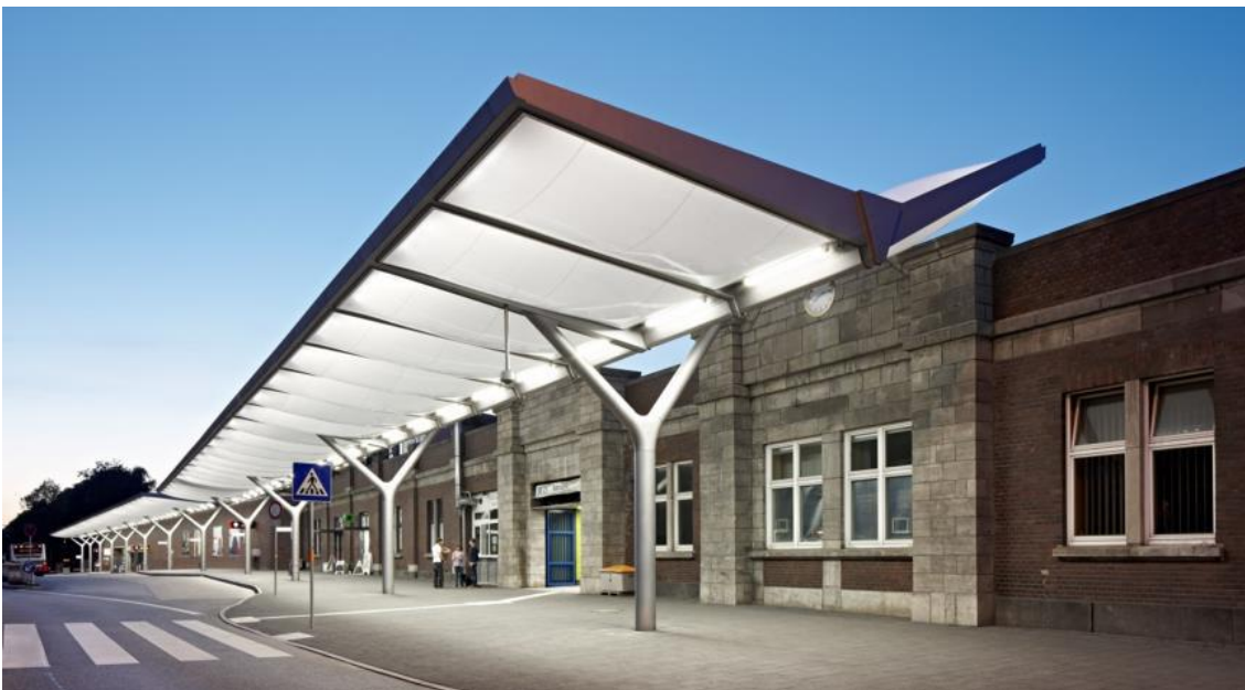
Figure 2: Bus Terminal Hamburg Barmbek [archimage Meike Hansen]
