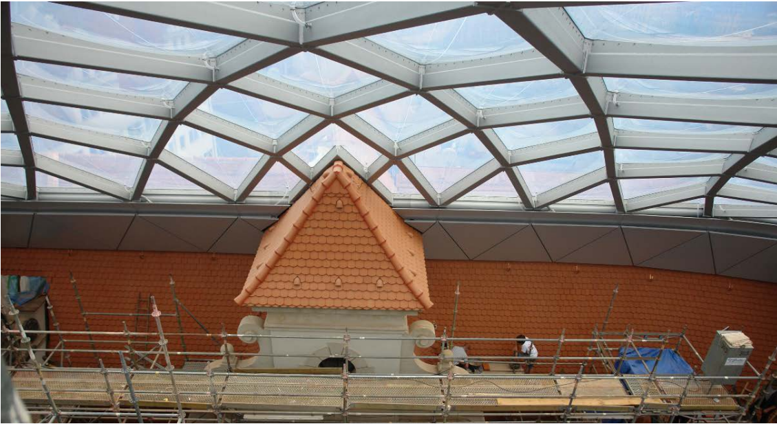
Figure 7: steel grid with cushion cladding [formTL]
