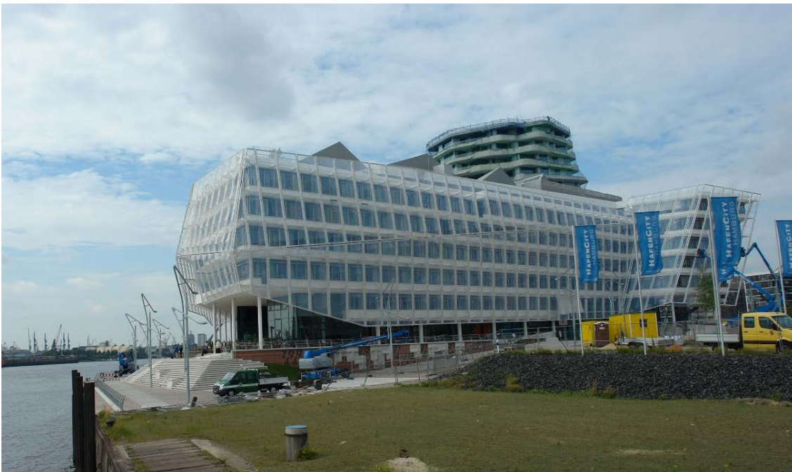
Figure 4: Unilever Hamburg, ETFE foil façade [formTL]
